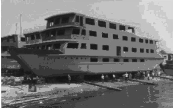
Figure 9. Vessel under construction.
