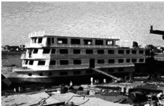
Figure 10. Vessel under construction.
