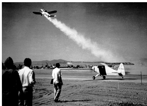
ROCKETRY TAKES OFF: In 1939, Malina's team received a small grant to develop jet-assisted takeoff rockets for the U.S. Army Air Corps. During flight tests in 1941 [bottom left], the JATO rockets cut the takeoff distance of a small civilian airplane by half; above, von Kármán is shown writing notes while Malina, to his left, looks on. Eventually, the group produced rockets with enough thrust to lift bombers like the Douglas A-20 Havoc [top left].
